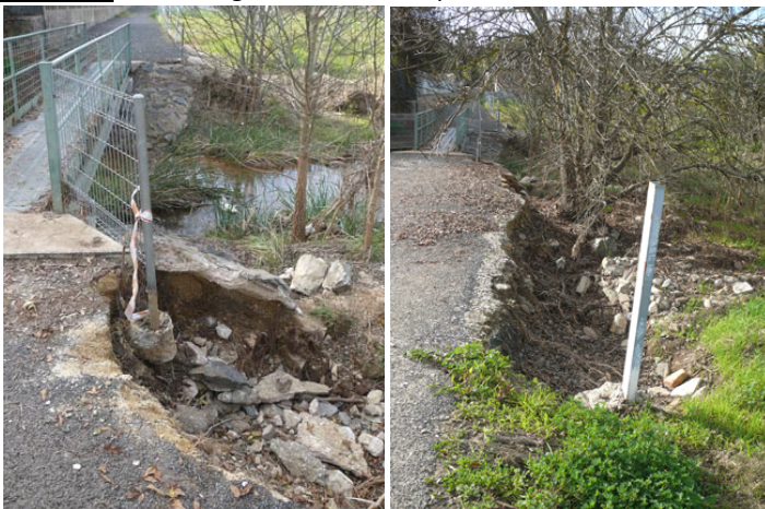
Possum Track Bridge abutments
